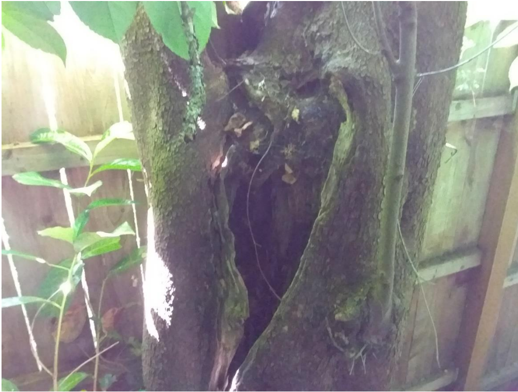
Figure 3. Photo of the top of the decay column of the dogwood.
